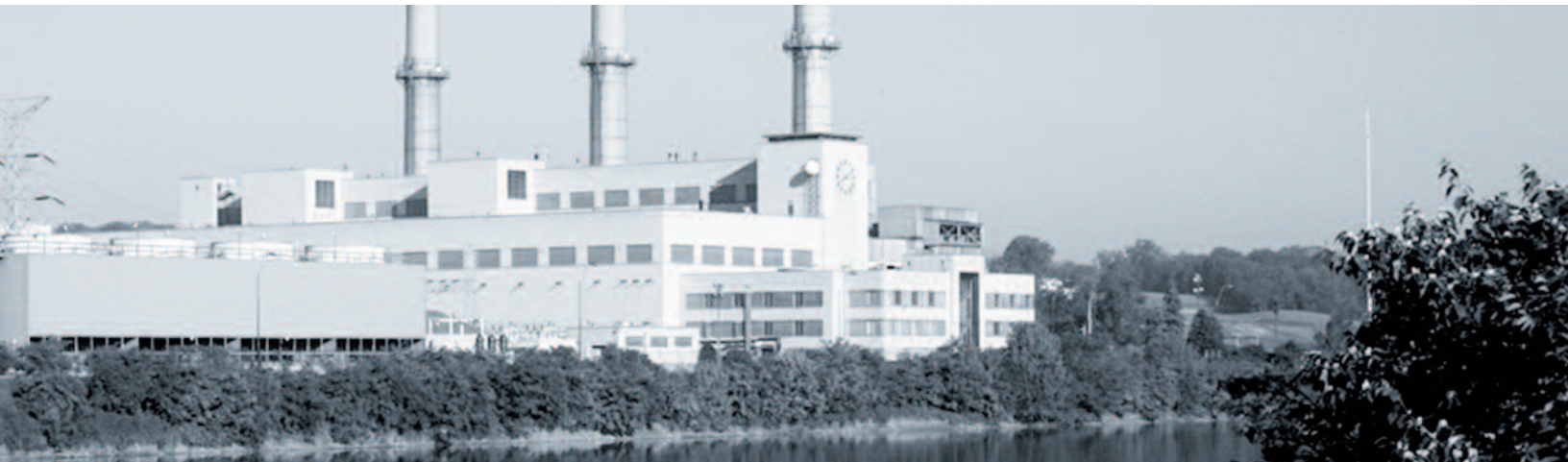
DP&L's Hutchings River facility. Photo courtesy of Dayton Power & Light Company
