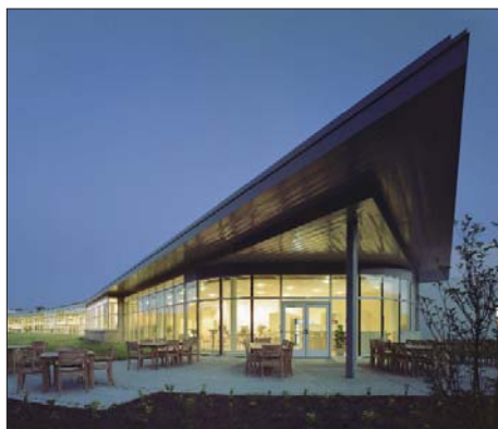
Air Liquide's recently constructed Research and Technology Center in Newark, Delaware is the eighth facility to join our network.
