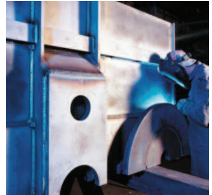
Heavy structure welding.
